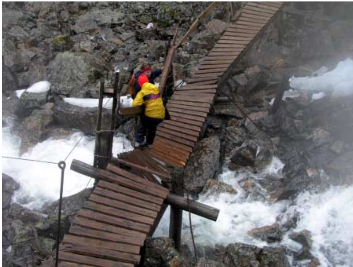
Figure 1 - Lack of maintenance can leave you hanging:
